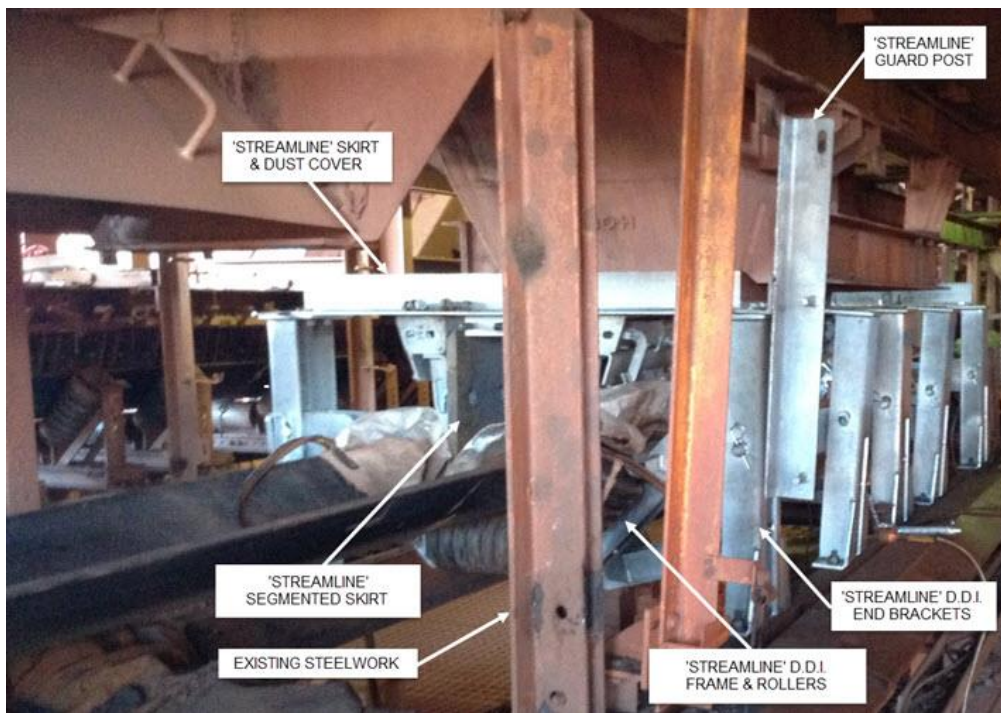
STREAMLINE CONVEYOR TRANSFER – INITIAL INSTALLATION
