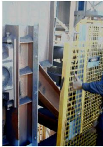
Installing DILO Guard
